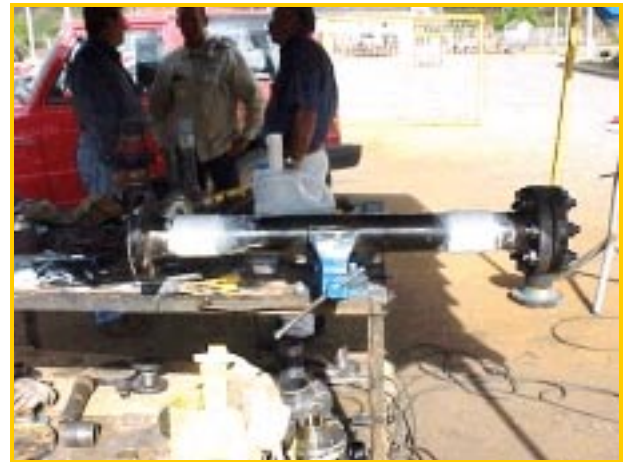
Figure No. 12 – Repaired and Completed Probe
