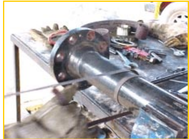
Figure No.2 - Cleaning of the Area for Defect "B"
