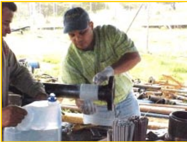
Figure No. 9 – Applying Syntho Glass® to Repair "B"
