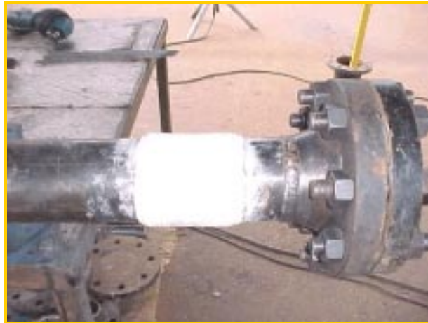
Figure No. 8 – Repair to "A" Completed
