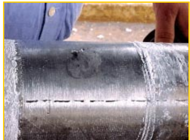
Figure No. 17 - Defect "A" after Removing the Syntho Glass Sleeve
