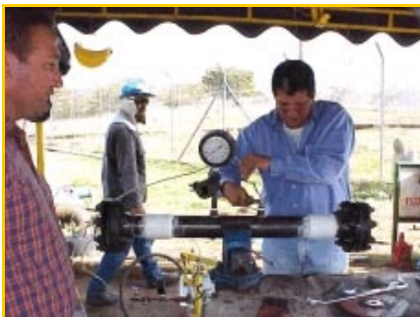
Figure No. 13 – Installing Pressure Gauge and Pump
