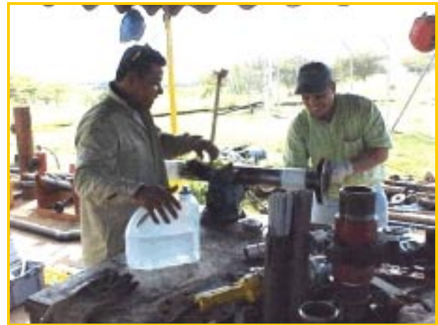
Figure No. 10 – Applying Syntho Glass® to Repair "B"
